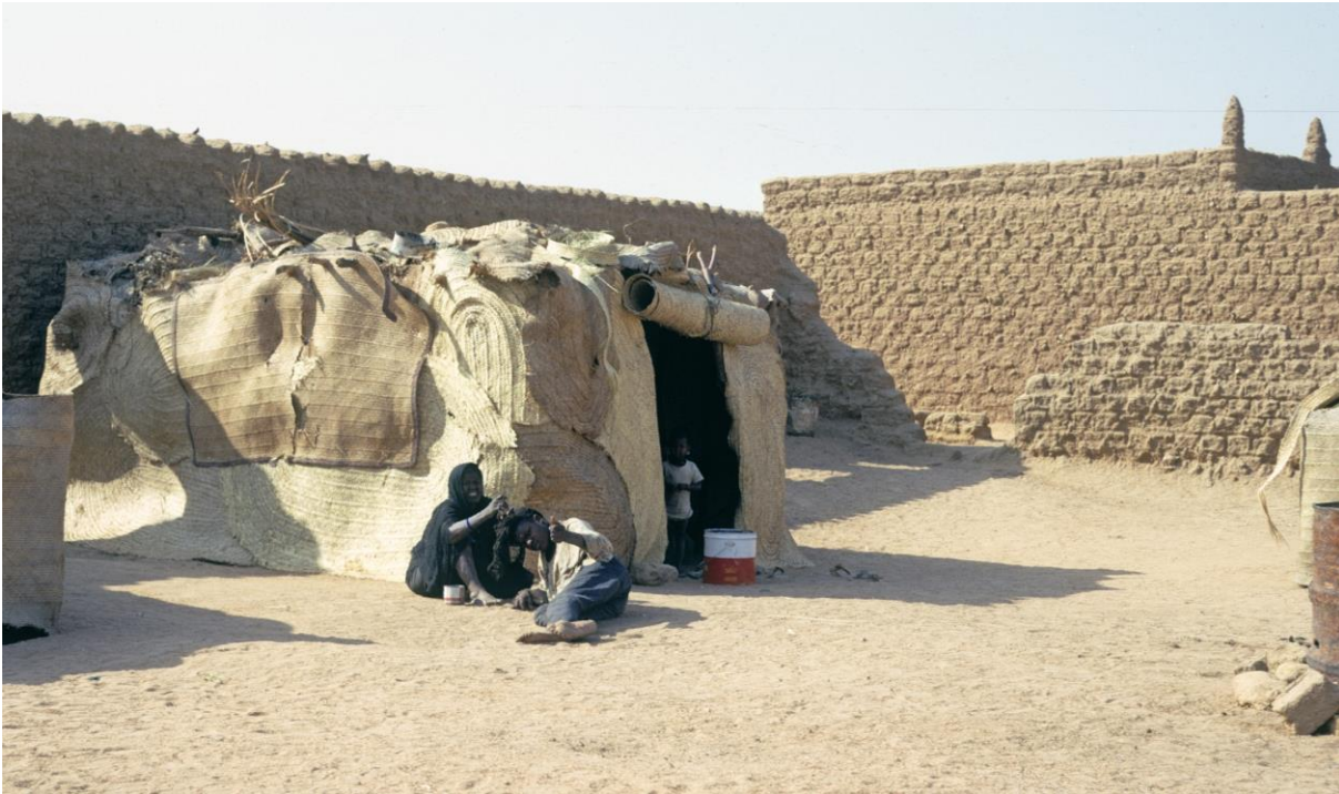
Fig. 2: Hamid Kumama's workshop is located inside the enclosing wall of his courtyard next to the simple mud dwelling house. It is a simple hut built directly on the mud floor. The walls are made of large woven palm fibre mats. Since it practically never rains in Agadez, the walls and roof serve primarily to keep out the glaring Sahel light and to be able to optimally judge the fire and the glowing metal with the eyes at the workplace.
