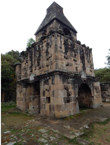
Figure 8.7: Blast furnace from the Mantasoa industrial complex of Jean Laborde (Credits: Vincent Serneels). Cast iron flowed through the furnace opening on the right. The opening on the left was connected to the hydraulic blower.
