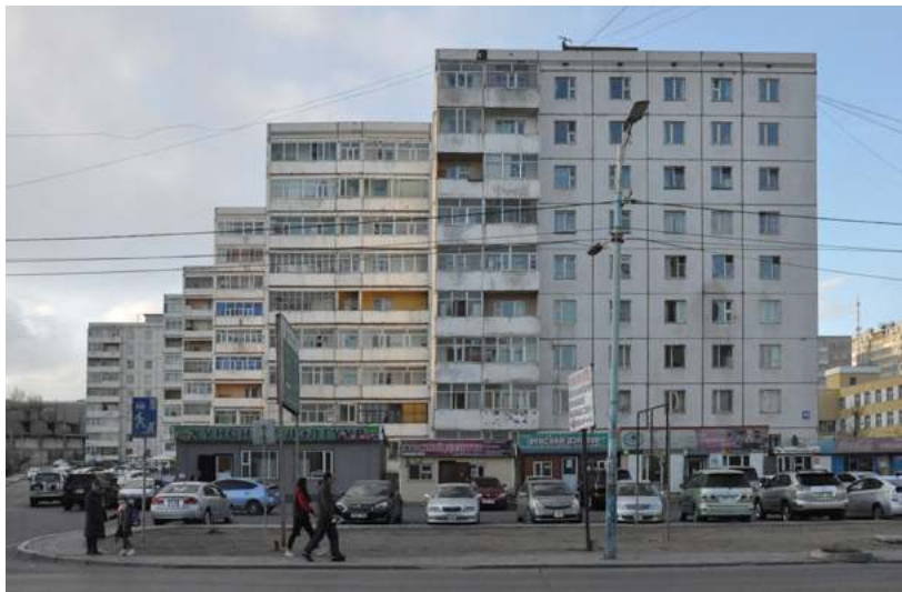
Figure 13: Residential buildings in the Gandan district, 1978-1983. Source: Photo by Łukasz Stanek, 2018.
