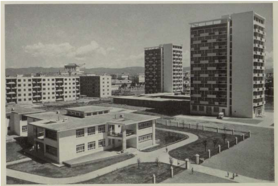
Figure 10: Mikroraiion 5 in Ulaanbaatar, with a kindergarten, 5-story residential buildings and two towers of Bayangol hotel. Gong Deshun, Beijing Industrial Design Institute (design 1964).
