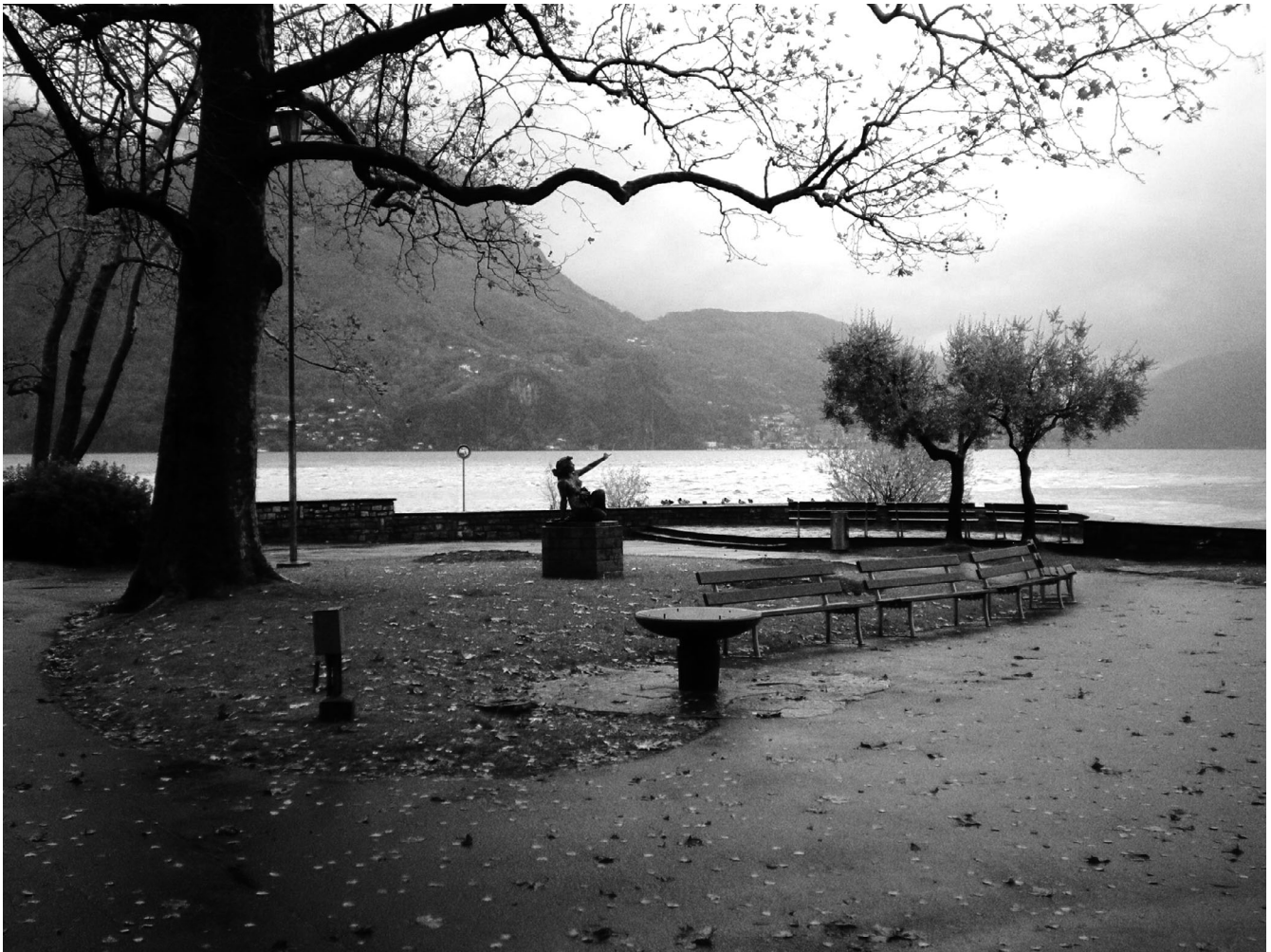
FIGURE 3 The rotunda before restoration.
