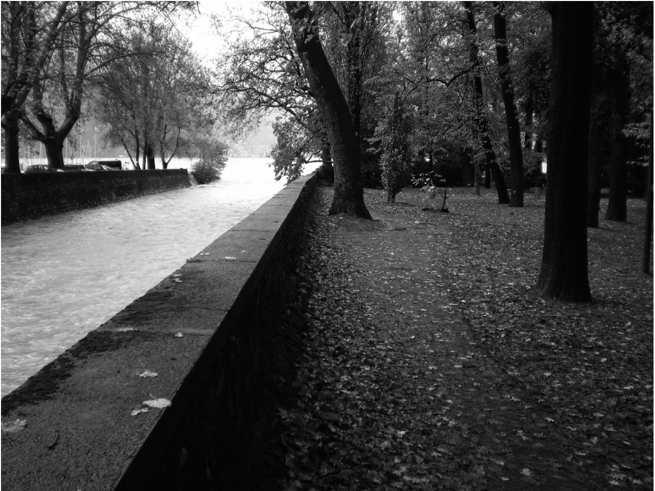
FIGURE 2 The Cassarate before restoration.
