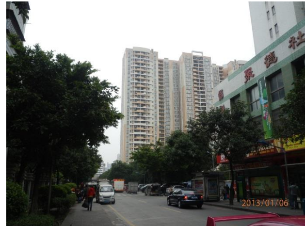
Pho. 5.4 Housing blocks in Jude community (Phase III)
