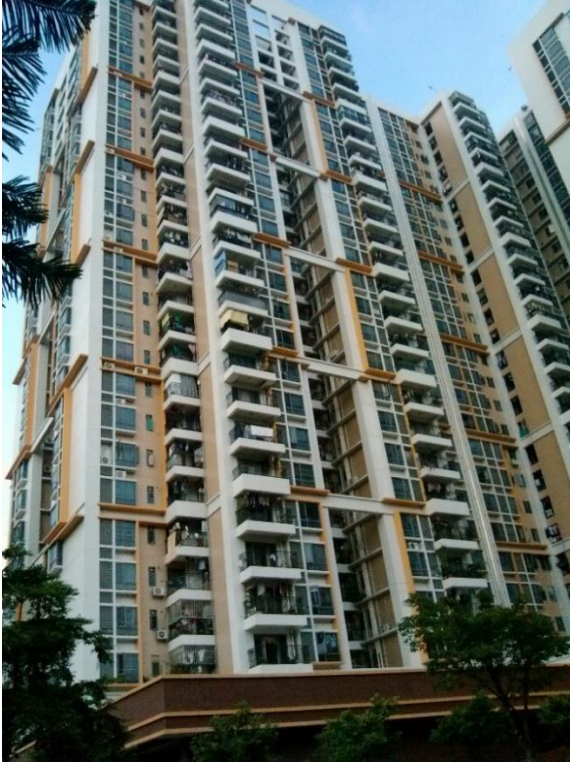
Pho. 5.25 Housing blocks in Tai'an community
