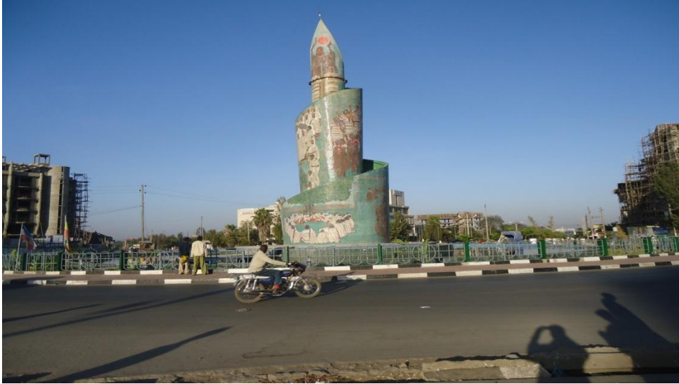
Picture 6: A monument completed with its length shortened.
