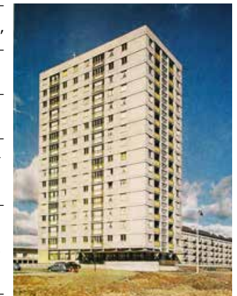
11 An apartment block constructed with Jean Baretts's patented prefabrication method: "Ville verte" of Canteleu by architects Louard and Lechevallier
