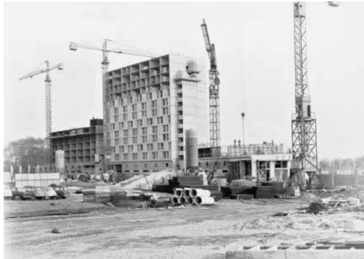
14 ZUP de Bayonne, construction of the high-rise blocks
